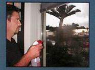
4. Peel clear backing to expose adhesive using two small lengths of low-tack tape at a corner of the sheet. Discard the clear backing and spray the adhesive side of WindowGrip with water & detergent solution.
