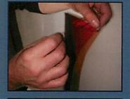
5. Apply WindowGrip using a hard rubber squeegee to remove water. Smooth with a clean, soft, lint-free cloth. Contact GAM for a 5" GAM rubber squeegee.
